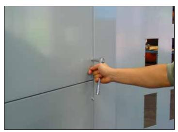
Figure 39. Removing the Bolts.
